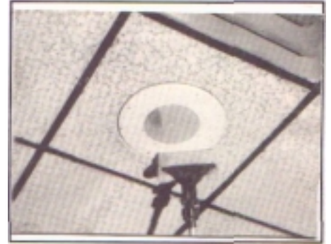
Ceiling grids/air conditioning vents/ speaker covers/light fixtures/sprinkler heads or any other plastic, metal, or glass item
